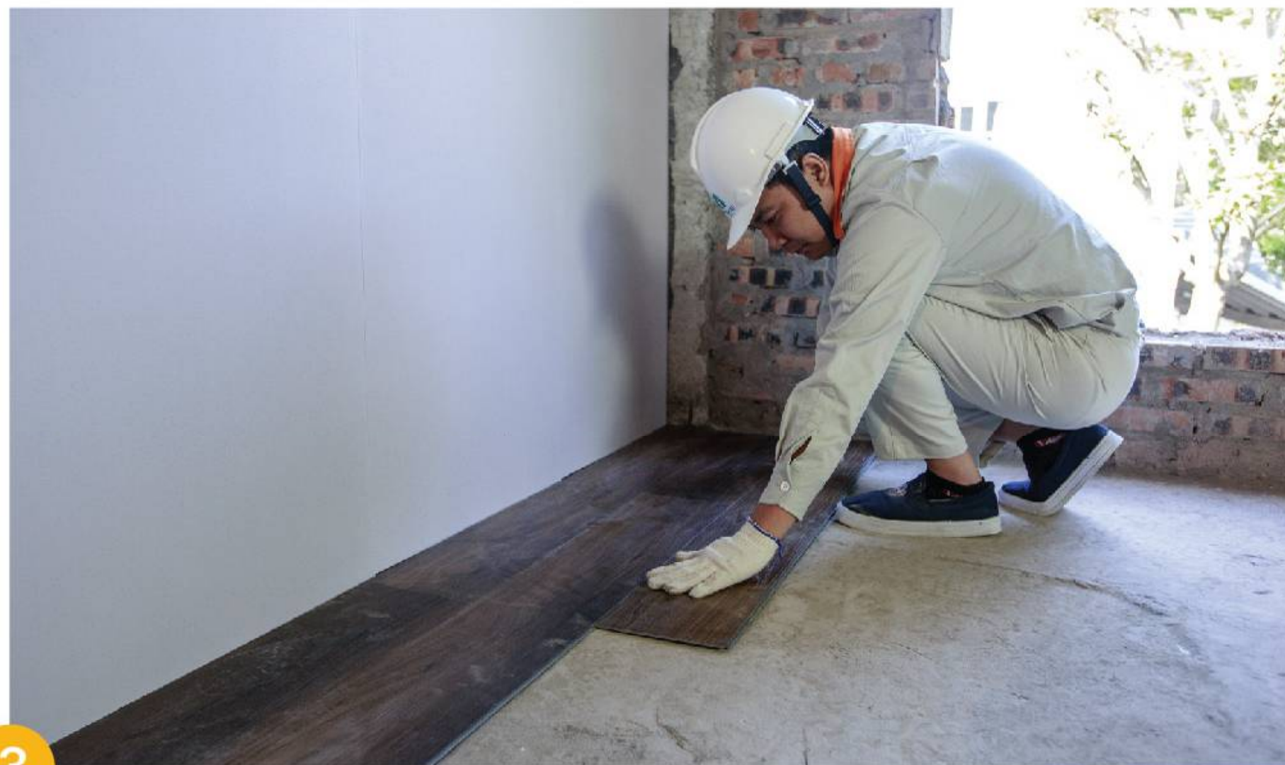
2 Step 2: Locate the first plank 3-5mm away from the wall. A multilayer design that includes underlayment will make it easier to install An Cuong flooring.
