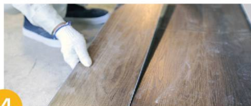
3 Step 3: Place the next plank to the first one according to the locking edge. Use a rubber hammer to tighten joints between the planks. Depending on the thickness of the flooring, add a pad to the floor edge before knocking to prevent breakage or deformation of the lock.
