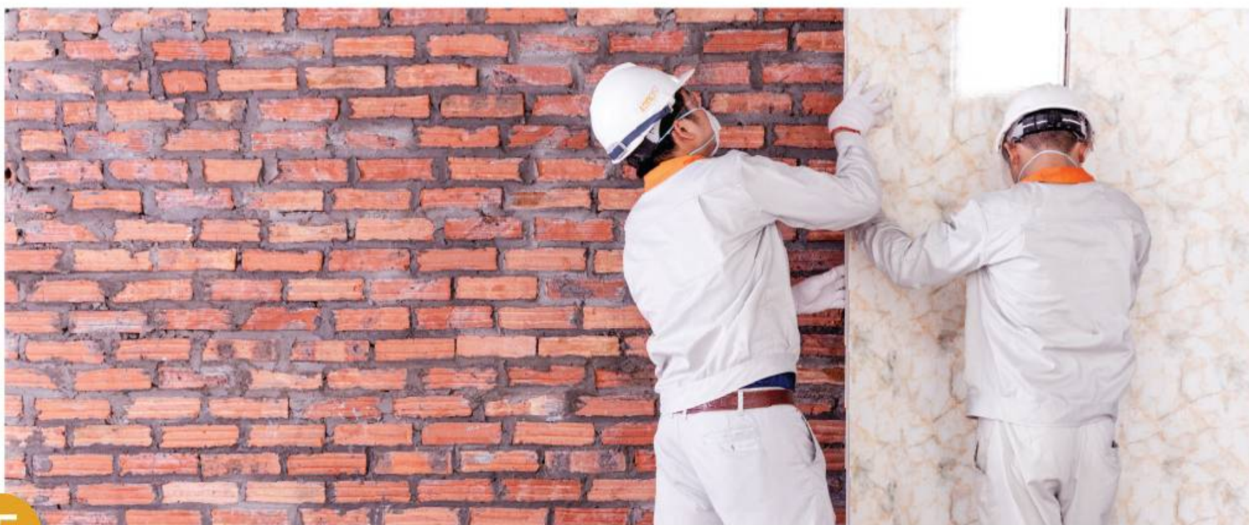
4 Put the hinged lock on the first plate, use a hatch or a nail gun to lock the hatch and the plate to the wall
